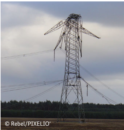
Storm damage caused by Hurricane Kyrill in 2007
